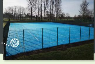
The team headed up north to Preston at the beginning of February to refurbish an existing block of tarmac courts covering 1,837m<sup>2</sup>. The first stage of the installation process involved drilling the base for drainage, jet-washing, then installing a Playrite 10mm shock pad and on top a MatchPlay 2 surface with inlaid lines for netball and tennis. Visually striking and a fantastic project to work on!
